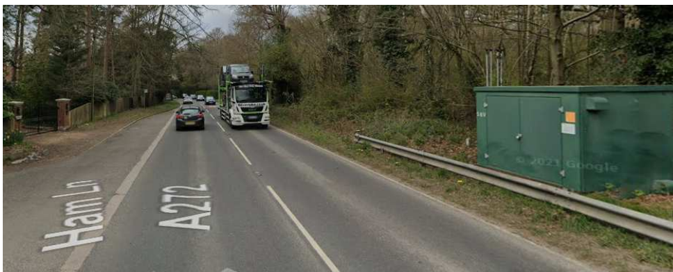
Figure 8.3 Gas kiosk on A272 opposite Ham Lane looking west
