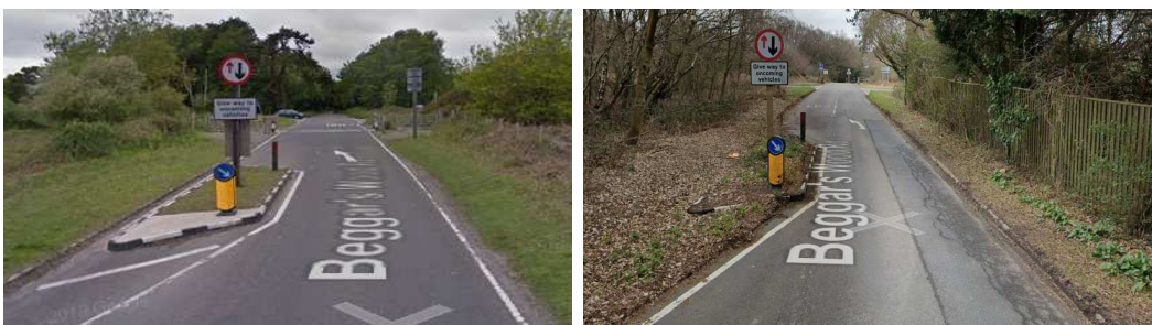
Figure 7.11 View of chicane traffic calming on Beggars Wood Road (speed limit 40 mph)
