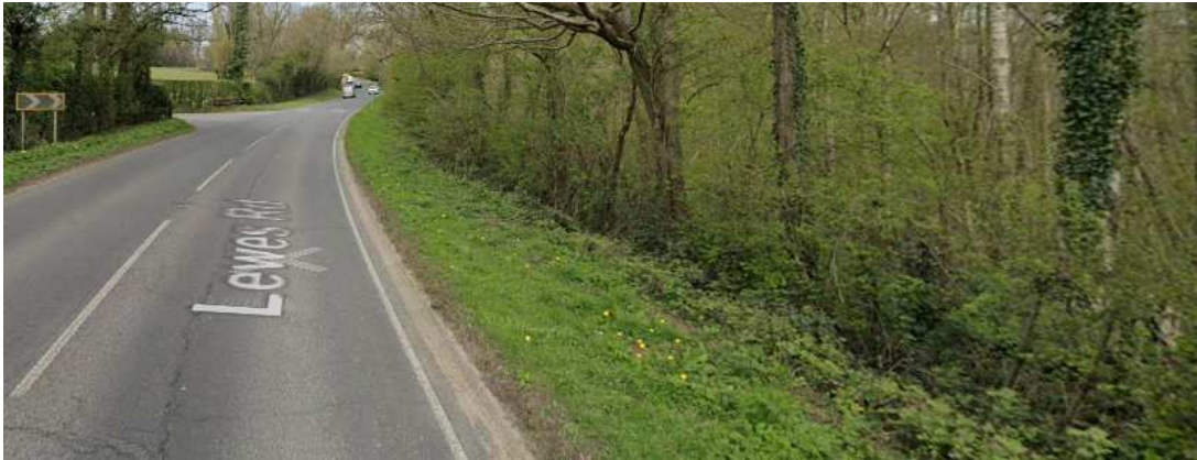
Figure 8.7 A272 adjacent to Cudwells land looking west - verge sloping away from road
