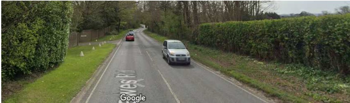
Figure 6.1 A272 looking east opposite Cudwells showing typical lane & verge widths
